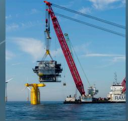
The components of the wind farm are transported to the site in large ships. They are installed at sea, using large vessels called jack-up barges or floating platforms with cranes capable of lifting very heavy loads. The offshore cable is installed using a special cable laying vessel.
